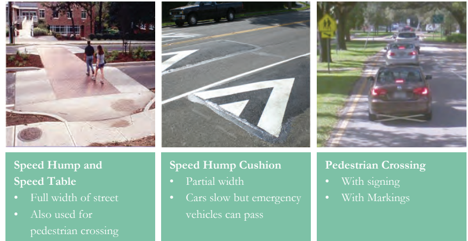
Figure 8.10: Pre-Approved Traffic Calming Devices
