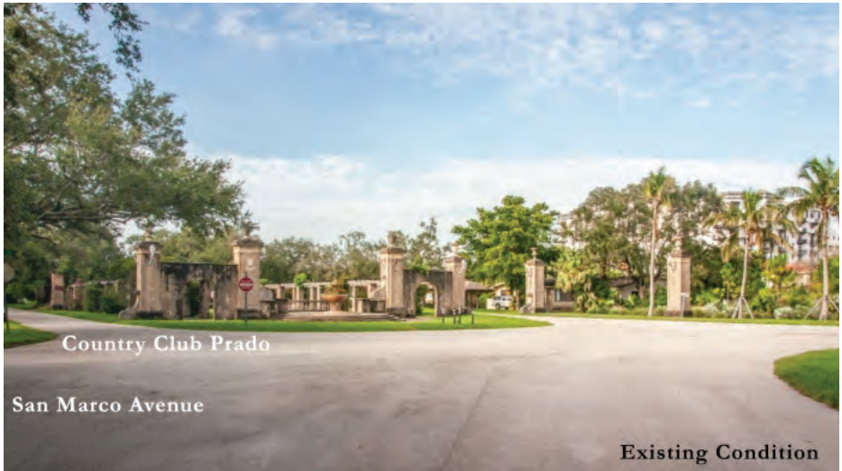
Figure 8.23: Country Club Prado at San Marco Avenue Concepts (Looking Southwest) – Preliminary Concepts
